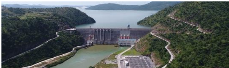
Figure 3: Aerial view of the Bui generation station
